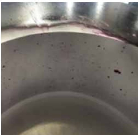
Fig 14a: Defective part excavated up to 135mm
